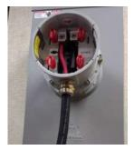
8 INSTALL METER SECURITY RING BETWEEN ADAPTER AND RESTORE-LITE® METER HEAD CORD SET
